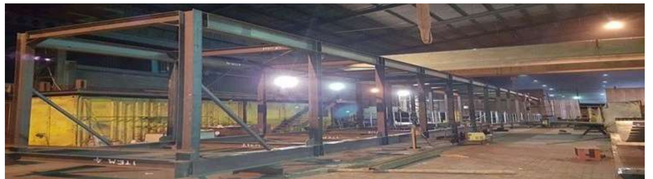
Trial fit-up of the bridge onto the outer feed-well
