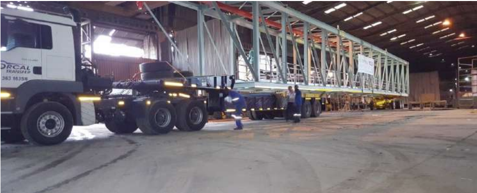
30 m bridge fully fabricated and transported in one piece
