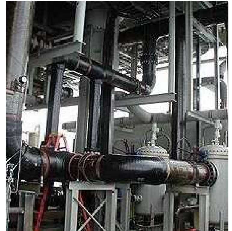
AECI Umbogintwini: Sulphur Plant Upgrade
