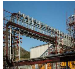
Barberton Tailings Plant
