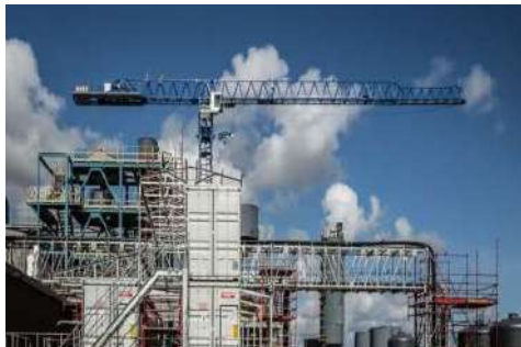
Barberton Tailings Plant: Erection
