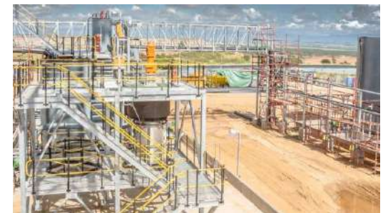
Sappi Ngodwana: Structural Steelwork
