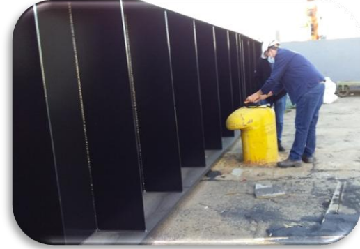
Lifting Platform Main Beams at Syncrolift Dry Dock in the Port of Cape Town
