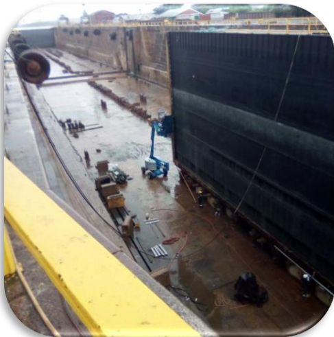
Rehabilitation of the Inner Caisson at the Dry Dock
