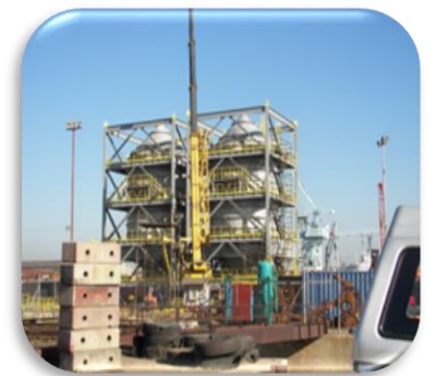
Built-In Modular Structures for Crystallizers for Nickel Mine
