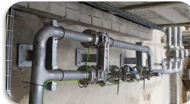
NPC Port Shepstone - Piping for Alternate Liquid Fuel
