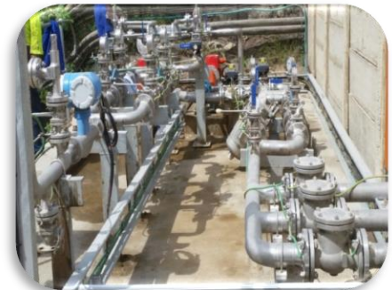
NPC Port Shepstone - Piping for Alternate Liquid Fuel
